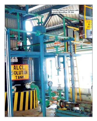
Figure 4: Fluoride Selective Ion Exchanger Operated At A Major Chemicals Manufacturing Company In Gujarat, India
